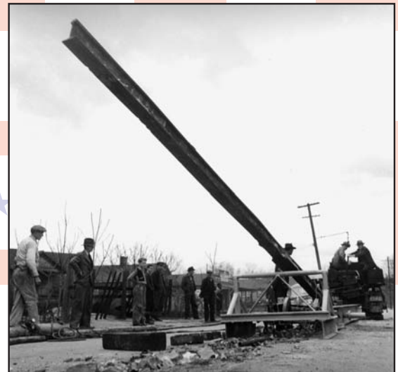
THE NEED FOR SCRAP METAL WAS SO GREAT THAT FOLKS SALVAGED MATERIAL FROM LANDFILLS AND PULLED UP TROLLEY RAILS BURIED UNDER PAVEMENT. THE TRACK BEING PULLED UP HERE RAN ALONG PATTON AVENUE.
